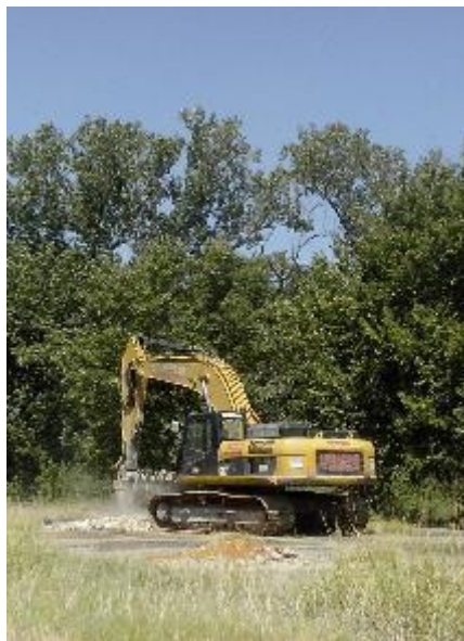
Construction begins on the $6MM Uplift Charter School
